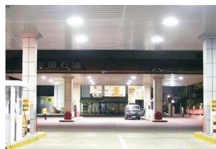
A Gasoline Station lit up with LED Bulbs
